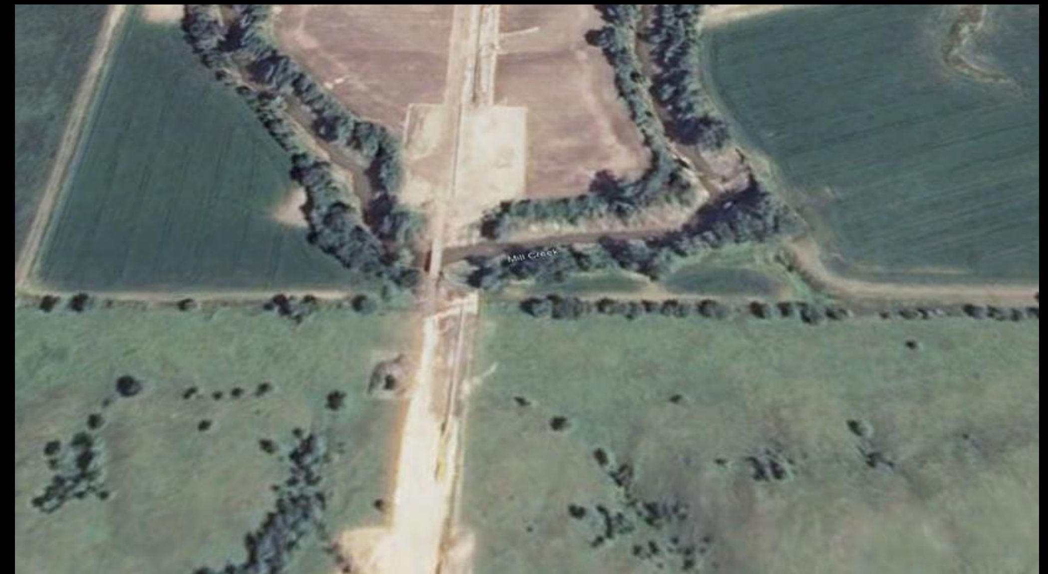
Figure 1: Mill Creek high resolution imagery from 2010 (credit USDA) showing the construction of the TC Energy pipeline.
